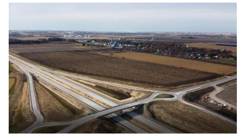
CSAH 3 View Northwest
