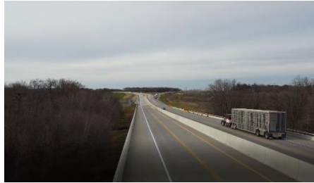
Hwy 14 Interchange Connection Looking West
