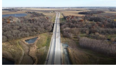
Hwy 14 Interchange Connection Looking East
