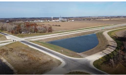
CSAH 1 View Northeast
