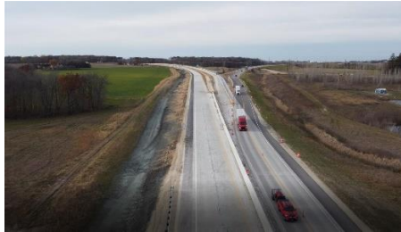
Hwy 14 Interchange Connection Looking West
