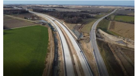
Hwy 14 Interchange Connection Looking West
