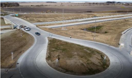
CSAH 3 View Northeast
